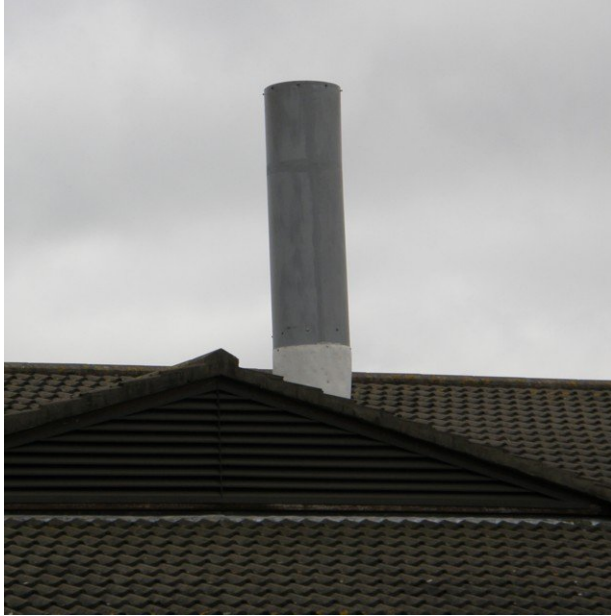
Transmitter Site Photo
