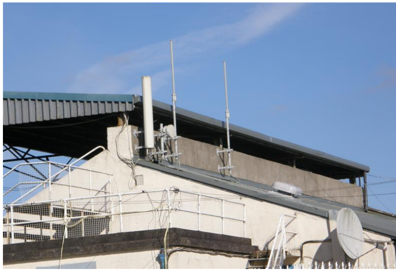
Transmitter Site Photo
