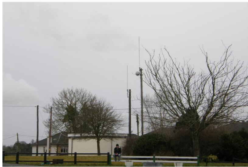
Transmitter Site Photo
