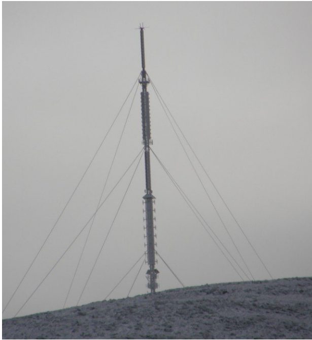
Transmitter Site Photo
