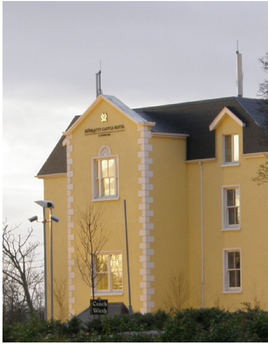
Transmitter Site Photo
