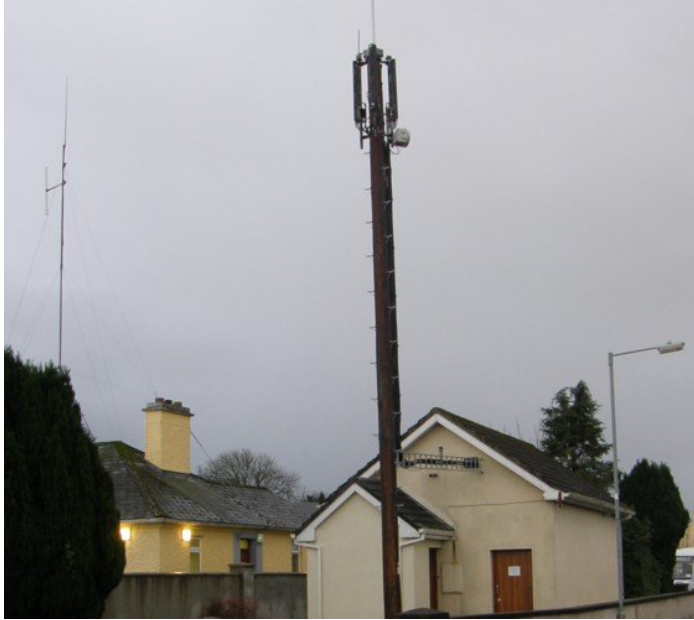
Transmitter Site Photo
