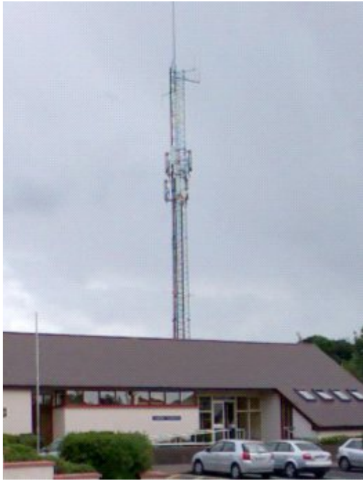
Transmitter Site Photo
