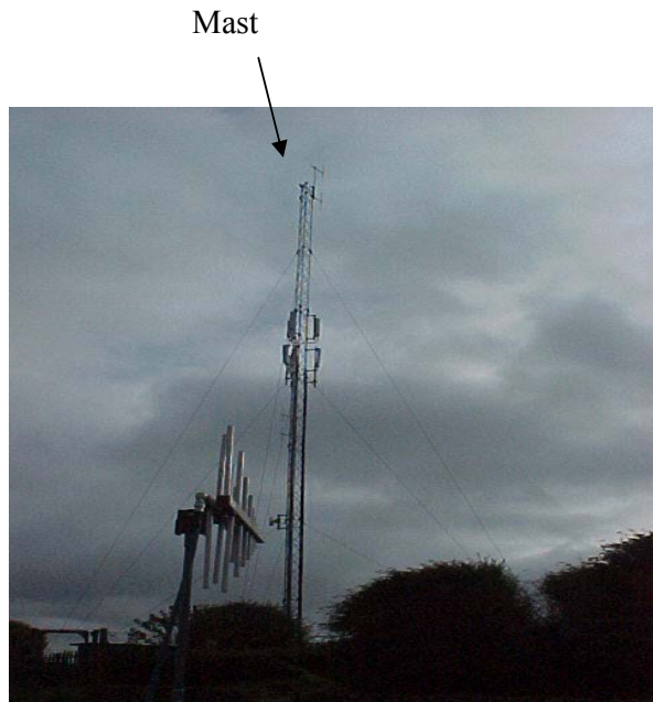
3.2.3.2 Position 2. Vinegar Hill. In passing bay on access road. 120m South-East of Mast.
