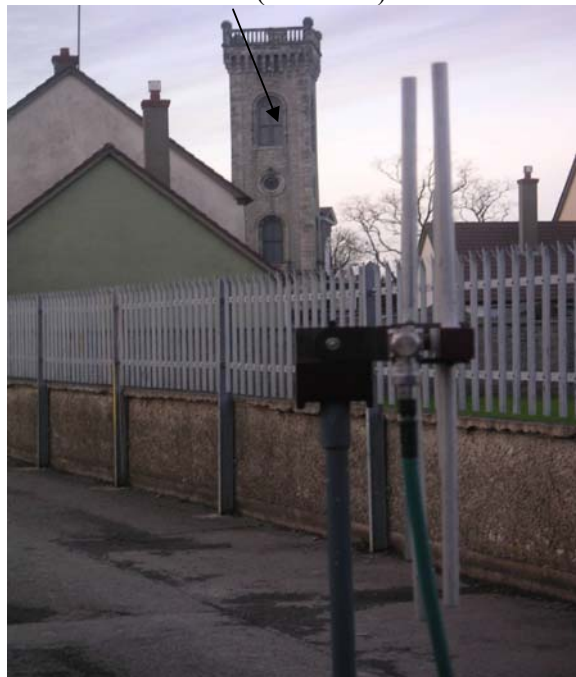
Mast (In Tower)
