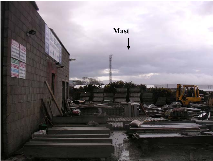
3.2.3.6 Position 6. Drumtracker, Forge Cross, B & F Building Supplies, in yard, approximately 200 m North of Mast.
