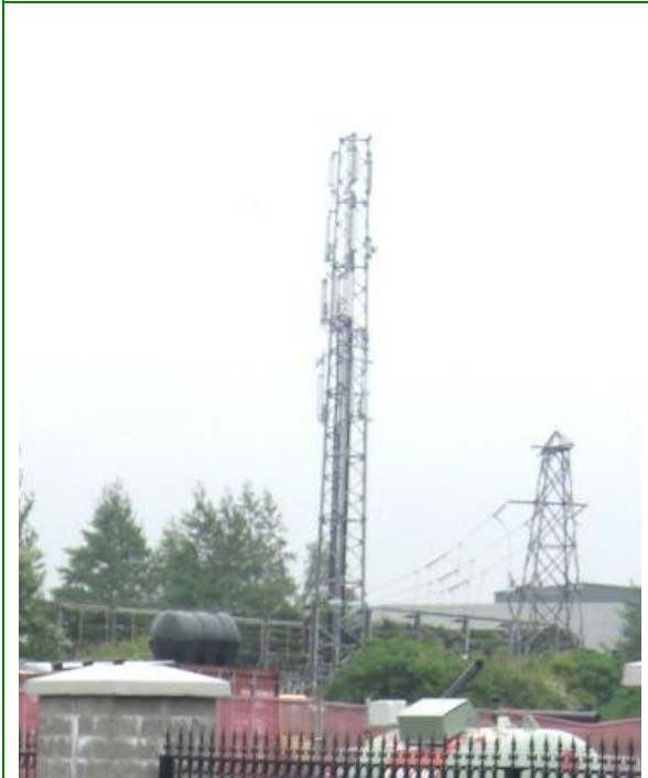
Transmitter Site Photo
