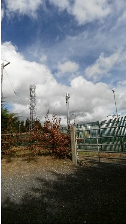
Transmitter Site Photo
