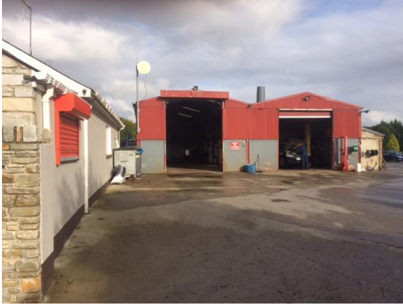
Transmitter Site Photo
