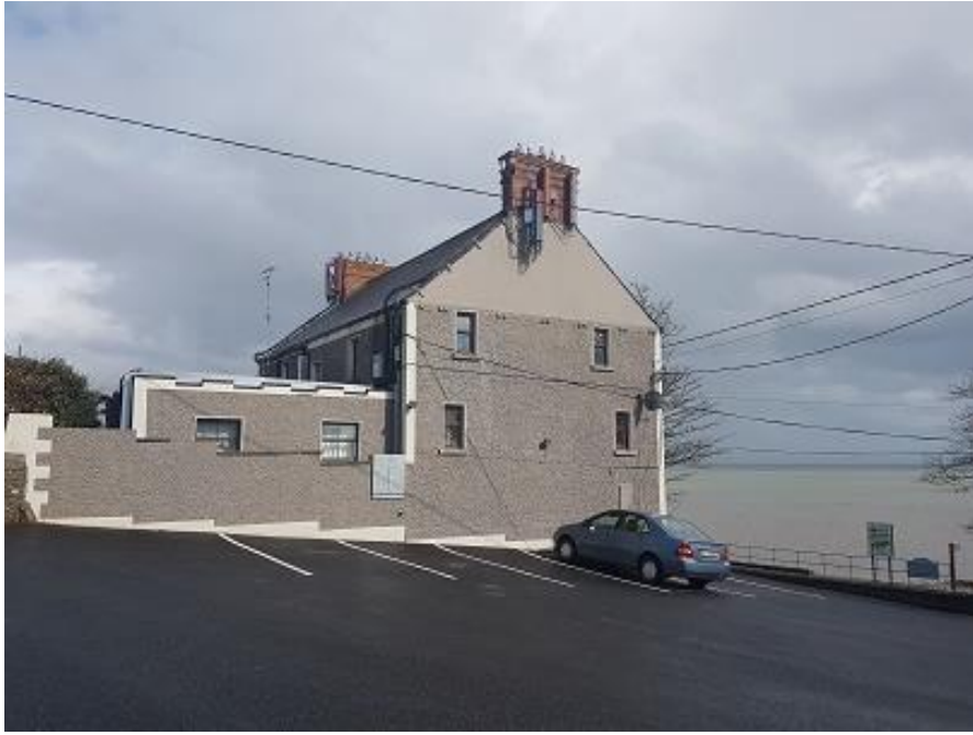
Transmitter Site Photo
