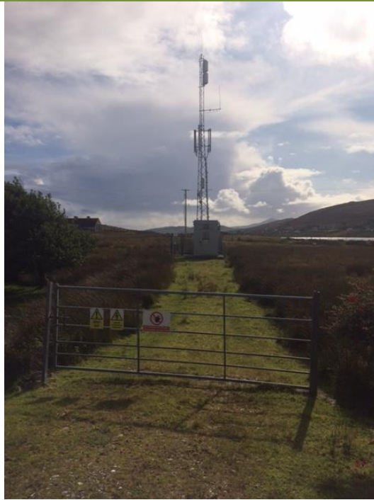
Transmitter Site Photo
