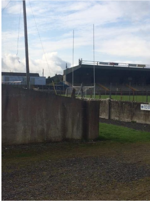
Transmitter Site Photo
