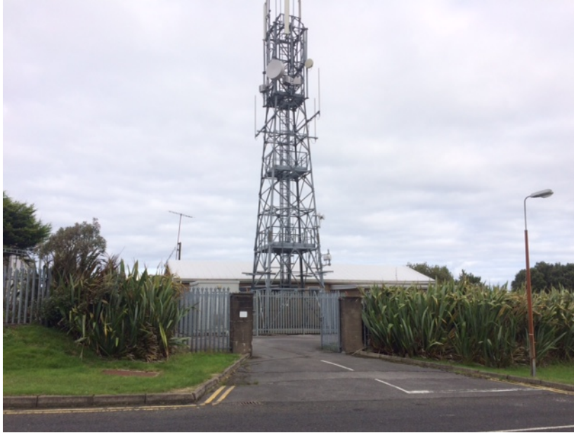
Transmitter Site Photo
