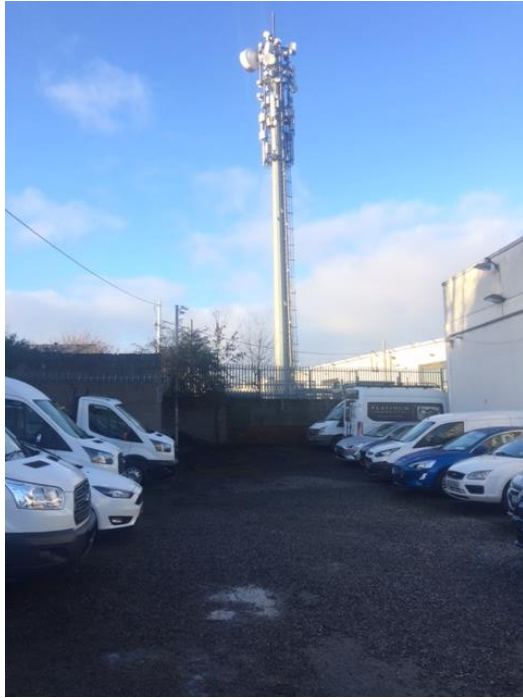
Transmitter Site Photo
