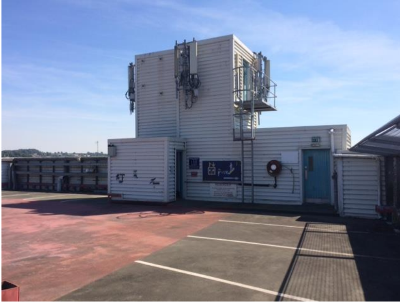
Transmitter Site Photo
