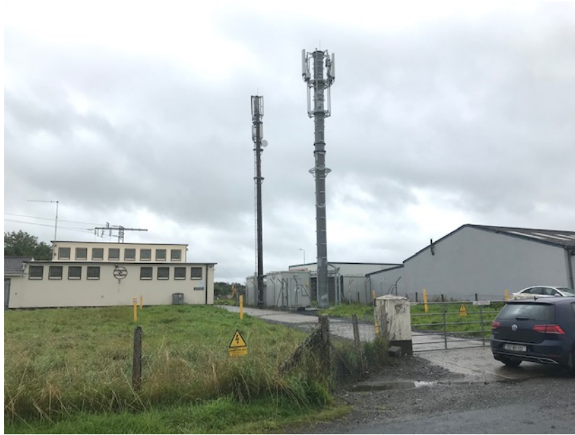
Designated Transmitter Site Photo
