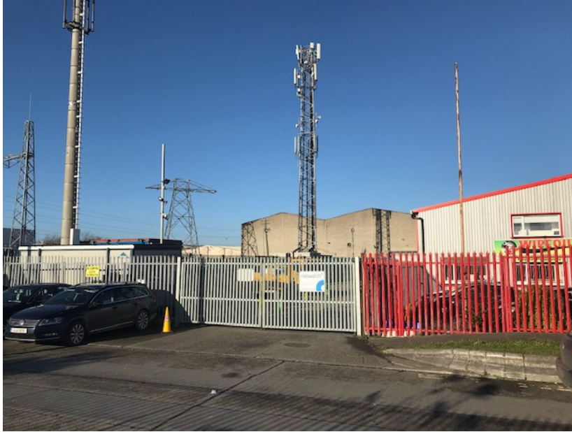
Designated Transmitter Site Photo
