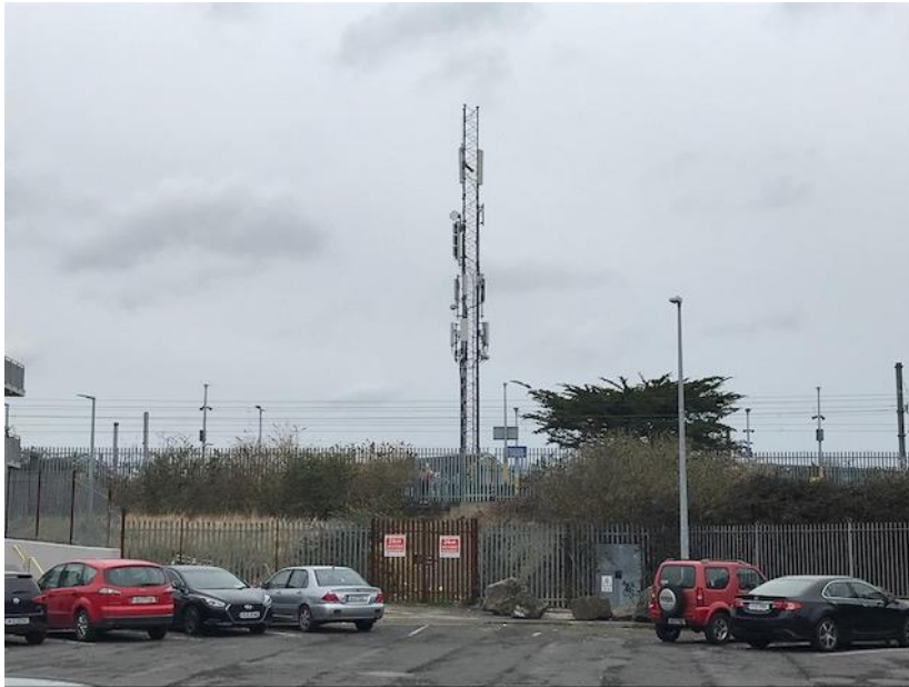
Designated Transmitter Site Photo
