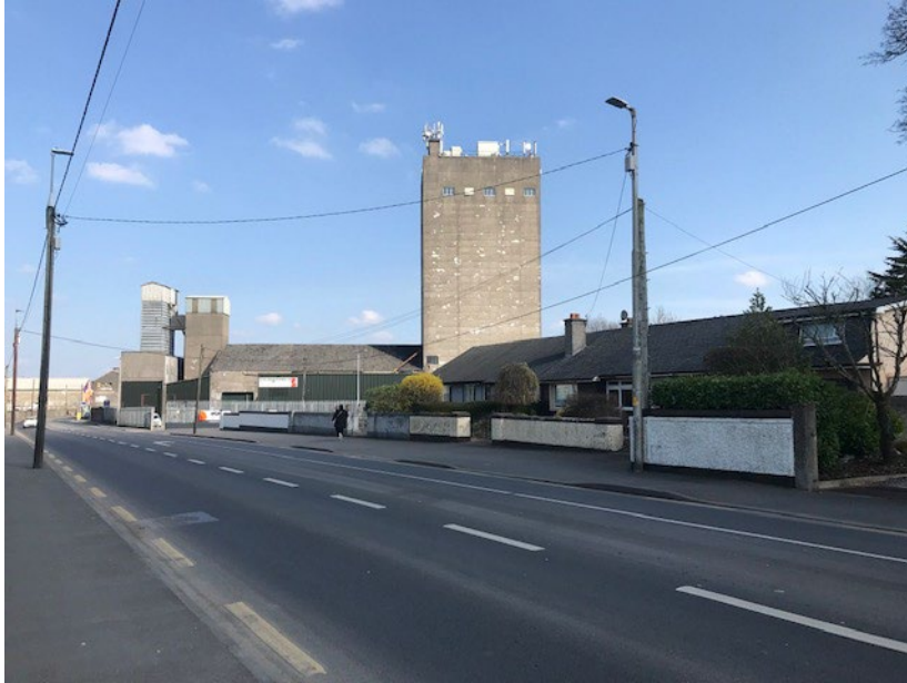
Designated Transmitter Site Photo
