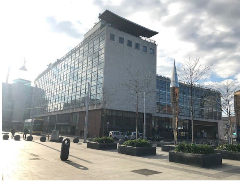
Designated Transmitter Site Photo
