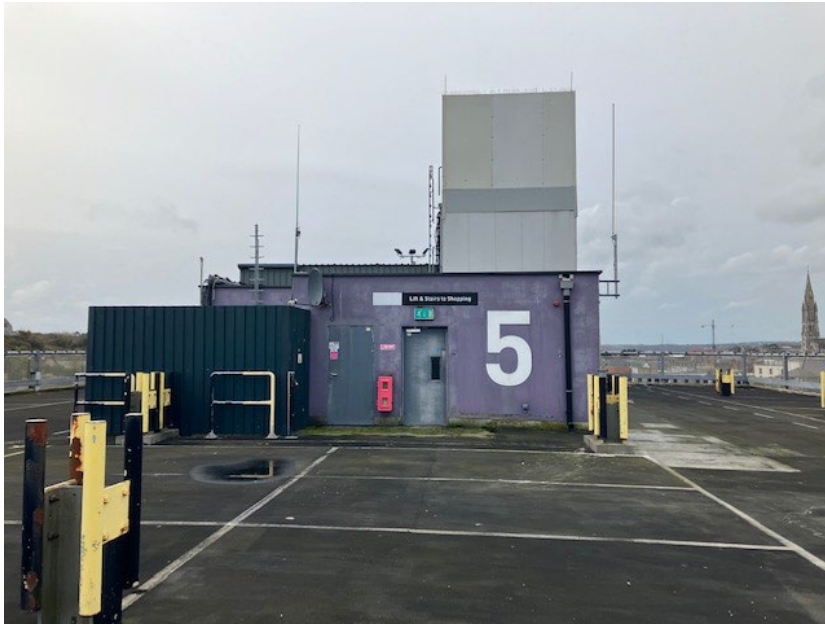
Designated Transmitter Site Photo
