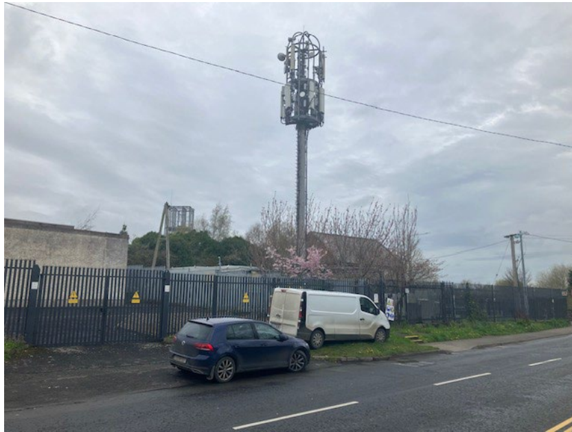
Designated Transmitter Site Photo
