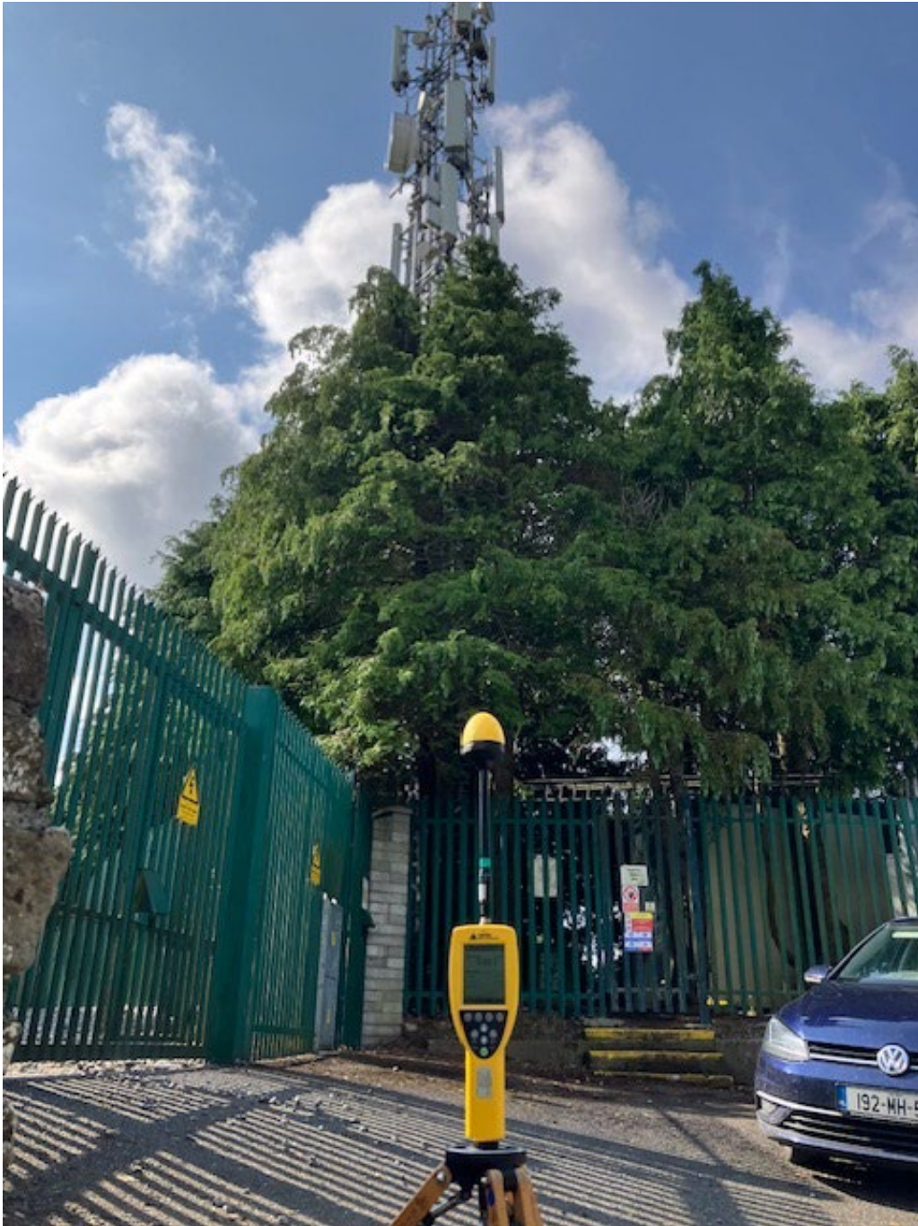
Photo 1. Broadband Measurement location looking towards antennas
