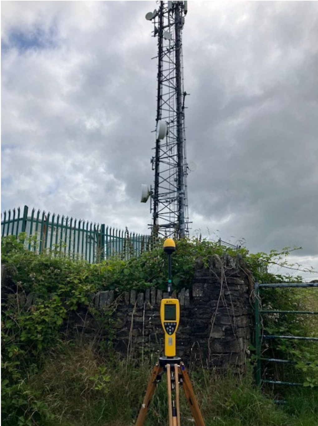
Photo 1. Broadband Measurement location looking towards antennas
