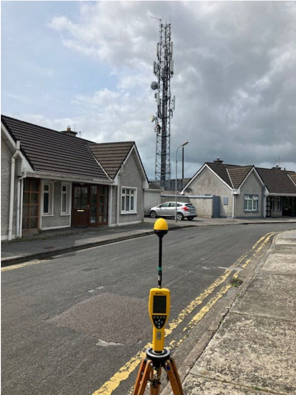
Photo 1. Broadband Measurement location looking towards antennas
