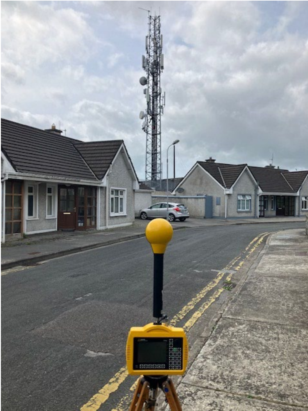
Photo 2. Frequency selective measurement location looking towards antennas
