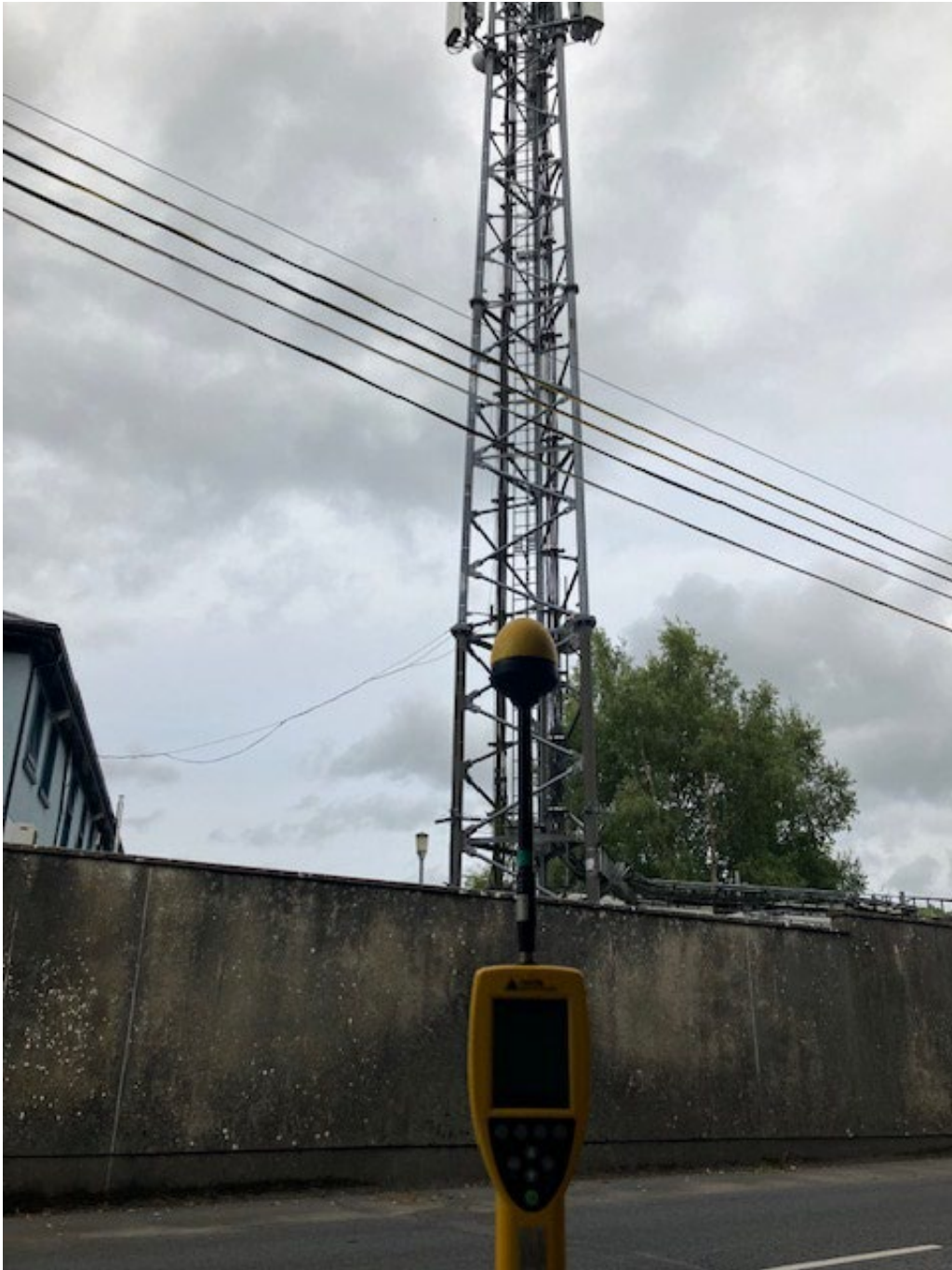
Photo 1. Broadband Measurement location looking towards antennas
