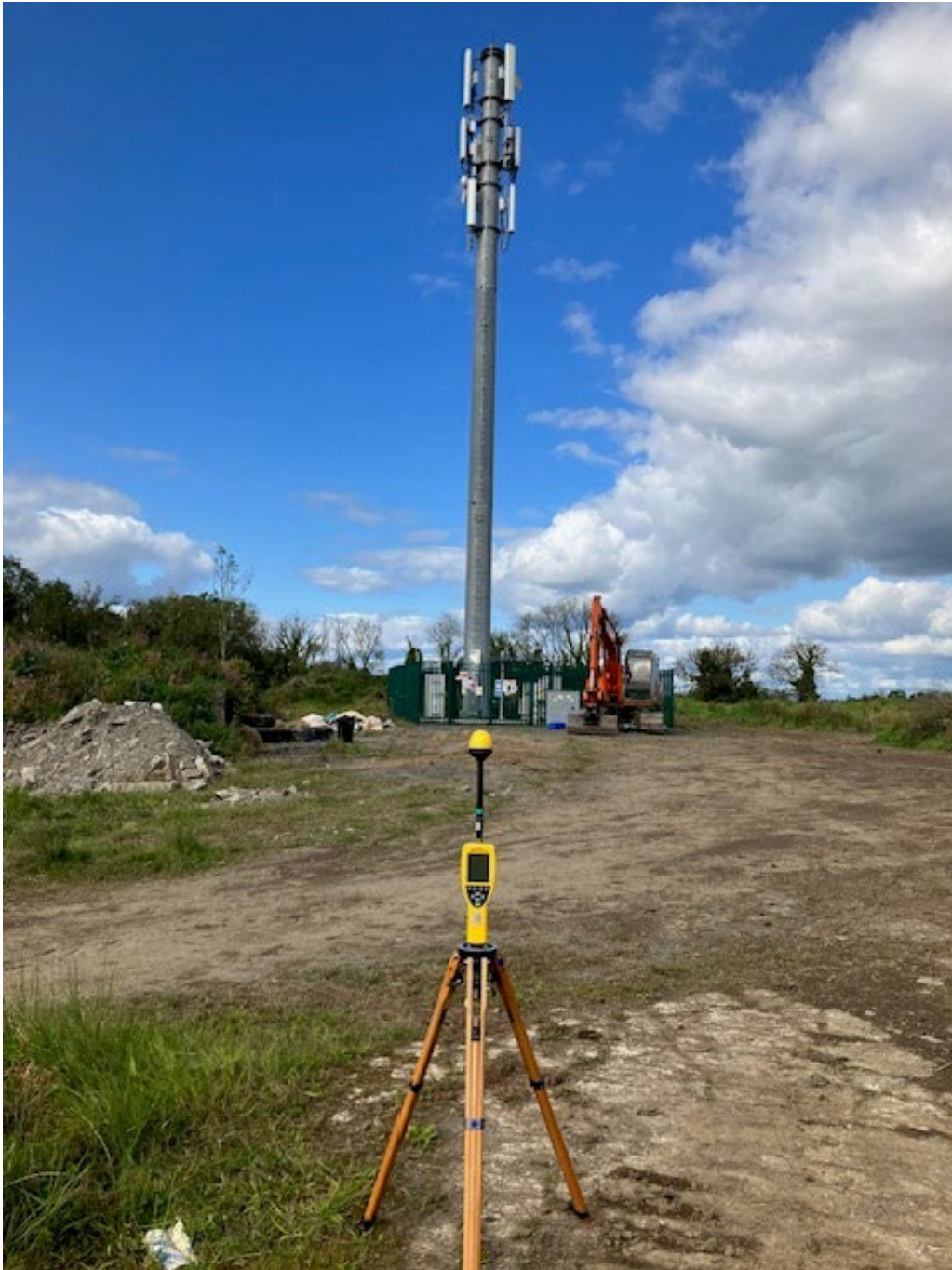
Photo 1. Broadband Measurement location looking towards antennas
