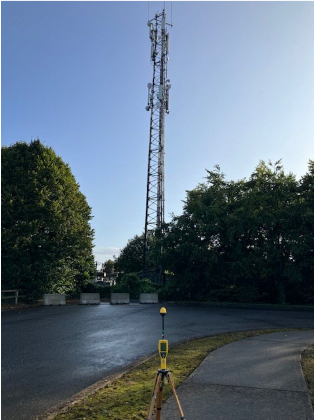
Photo 1. Broadband Measurement location looking towards antennas
