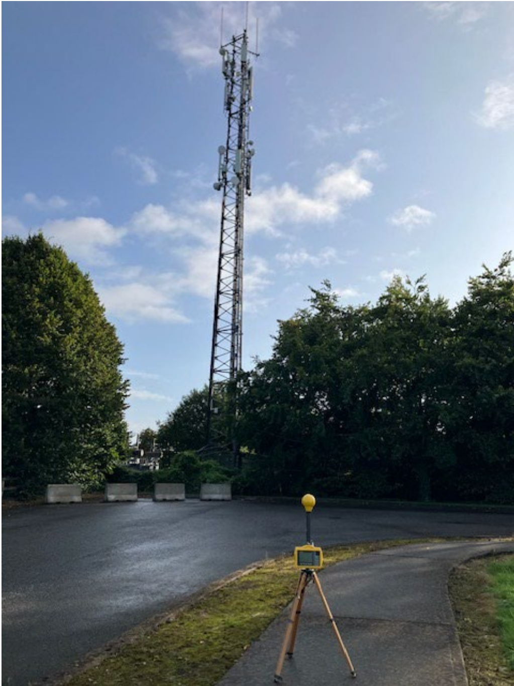
Photo 2. Frequency selective measurement location looking towards antennas
