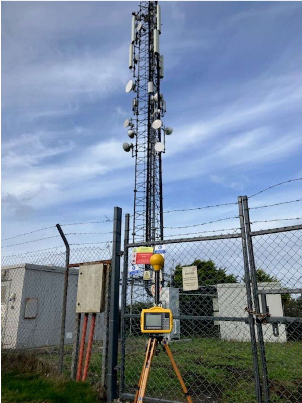
Photo 2. Frequency selective measurement location looking towards antennas
