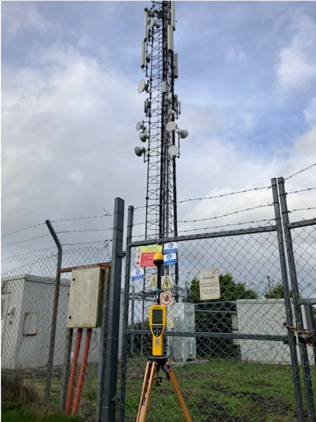
Photo 1. Broadband Measurement location looking towards antennas
