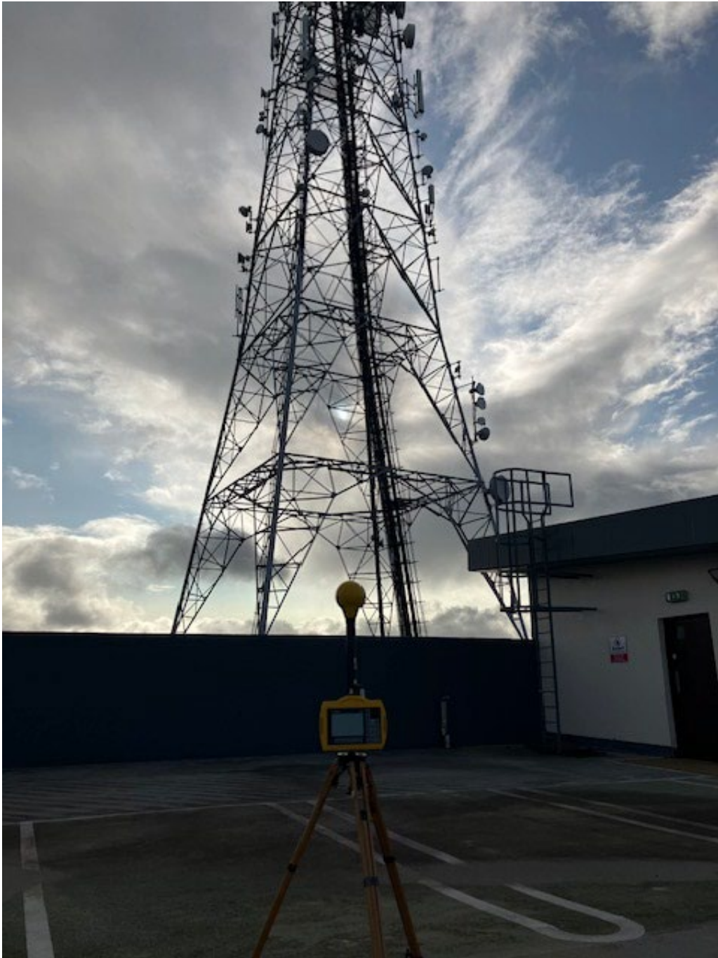
Photo 2. Frequency selective measurement location looking towards antennas
