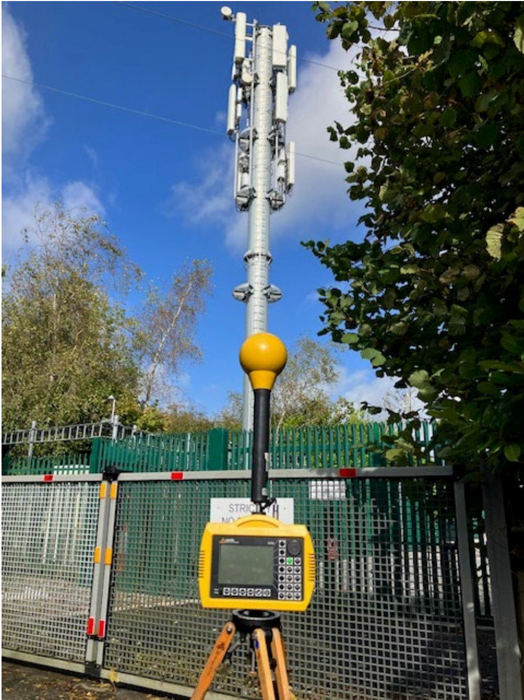
Photo 2. Frequency selective measurement location looking towards antennas
