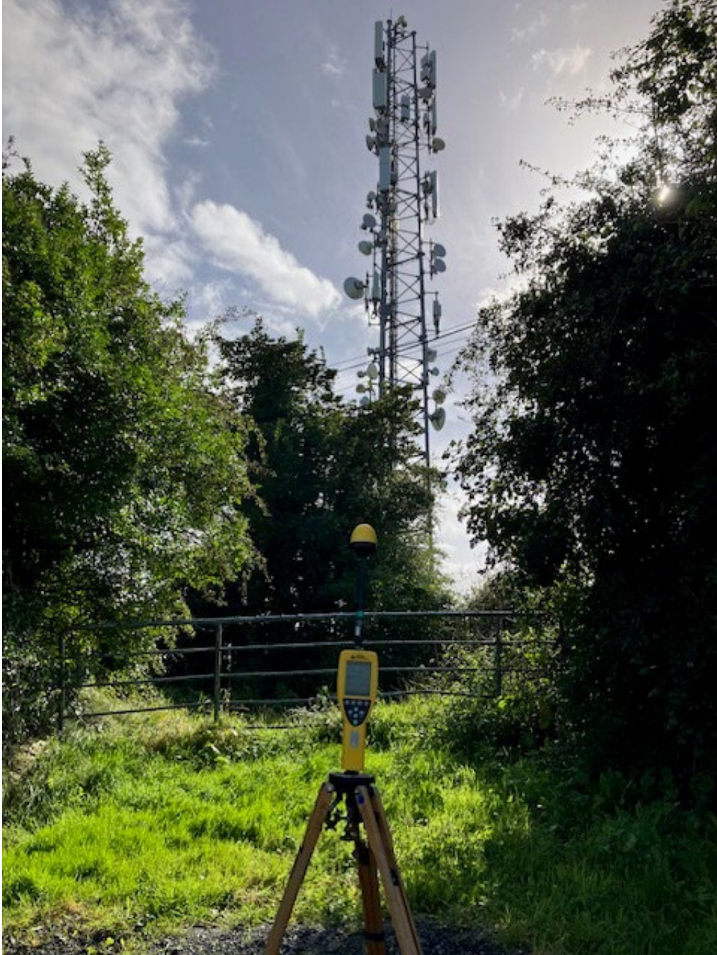
Photo 1. Broadband Measurement location looking towards antennas
