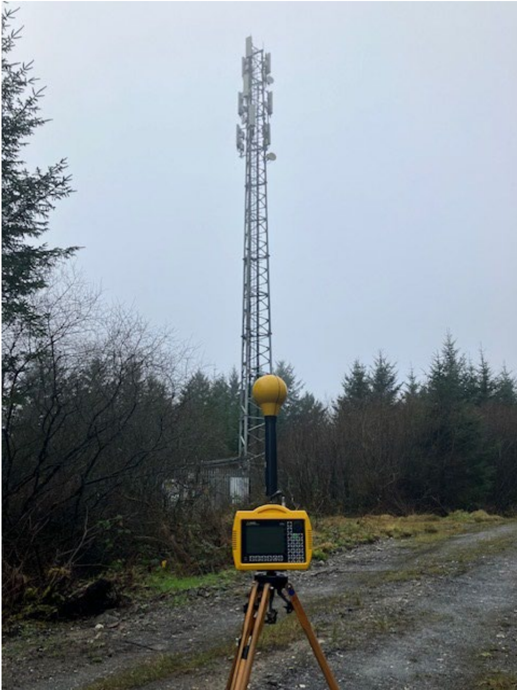
Photo 2. Frequency selective measurement location looking towards antennas
