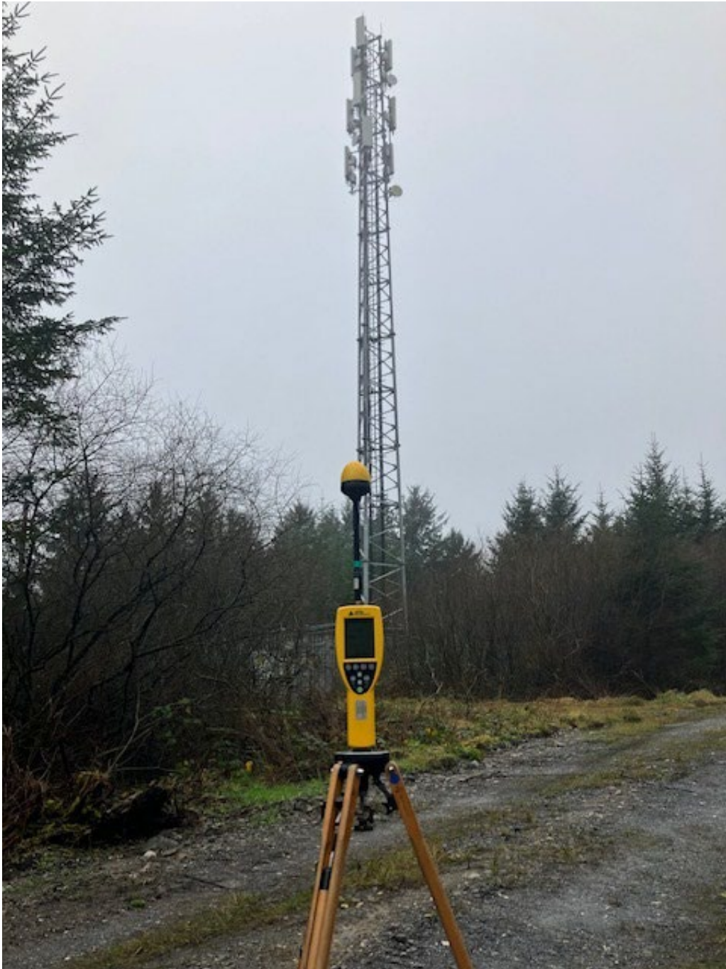
Photo 1. Broadband Measurement location looking towards antennas
