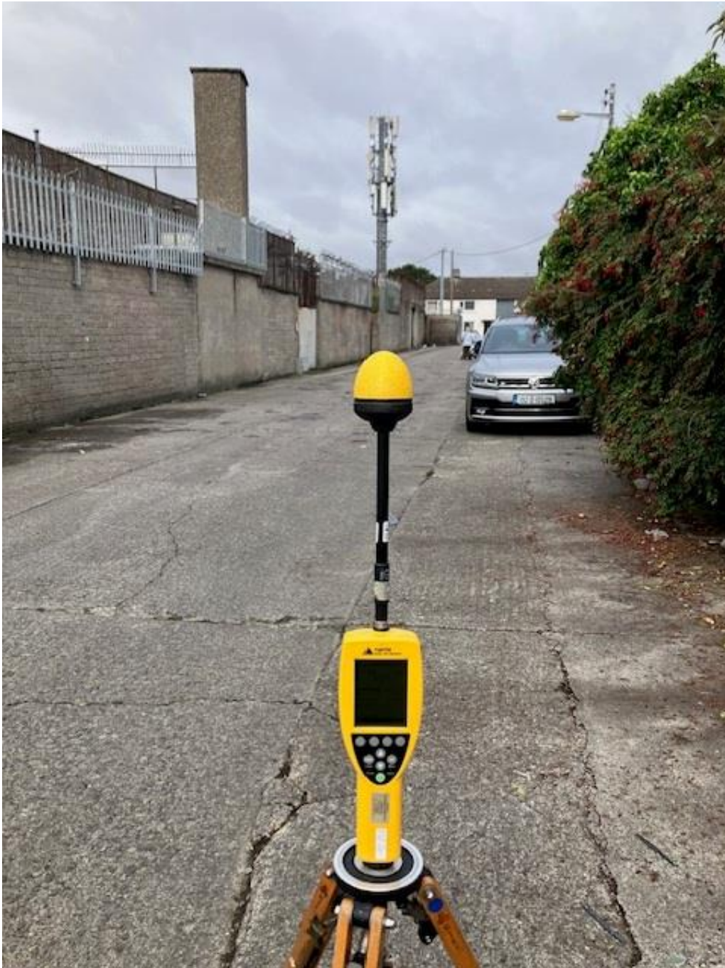
Photo 1. Broadband Measurement location looking towards antennas
