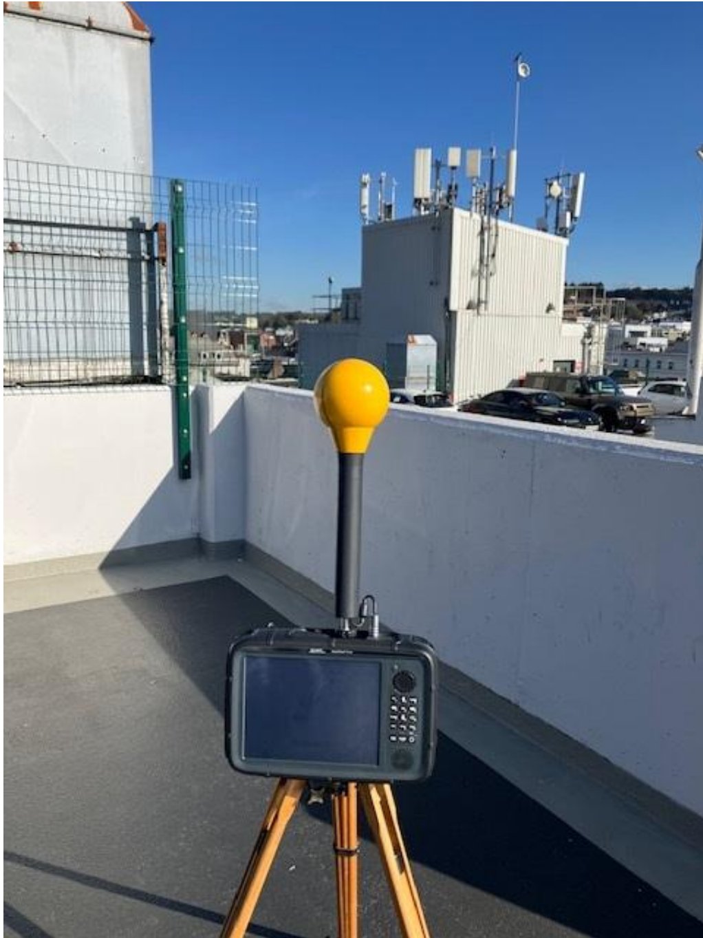
Photo 2. Frequency selective measurement location looking towards antennas
