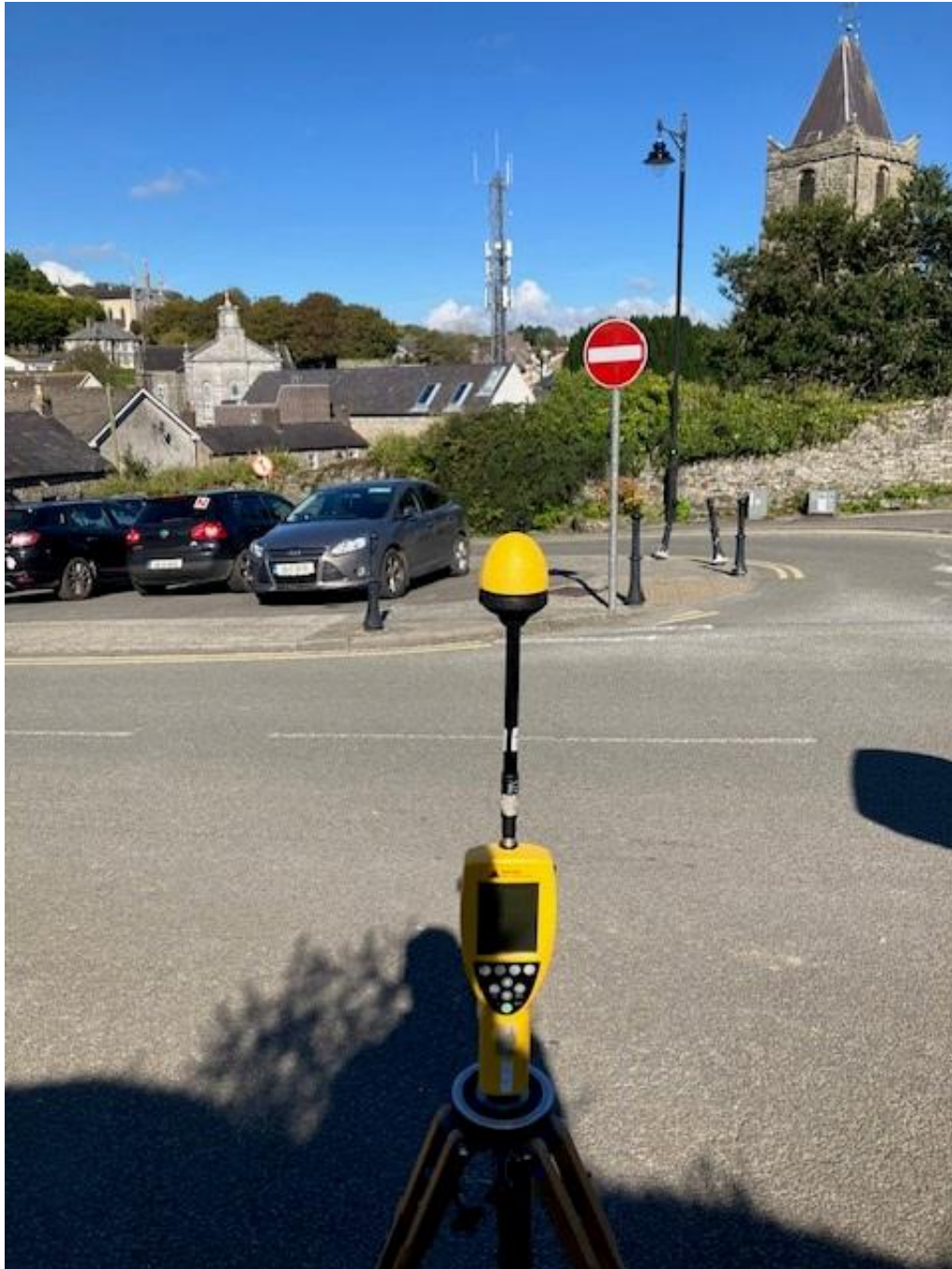
Photo 1. Broadband Measurement location looking towards antennas
