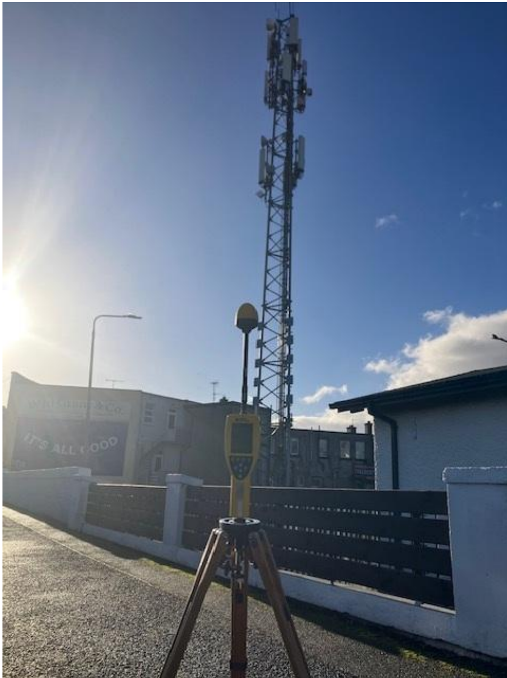
Photo 1. Broadband Measurement location looking towards antennas
