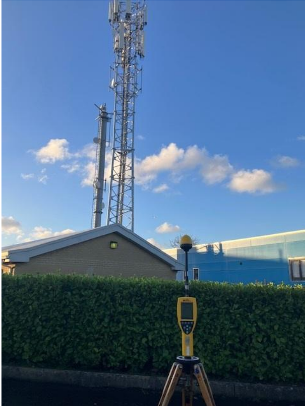
Photo 1. Broadband Measurement location looking towards antennas
