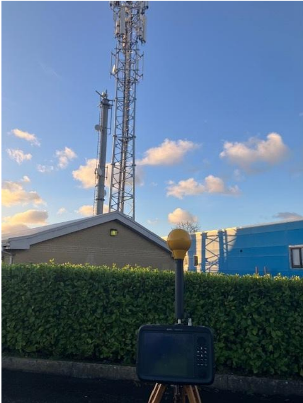
Photo 2. Frequency selective measurement location looking towards antennas
