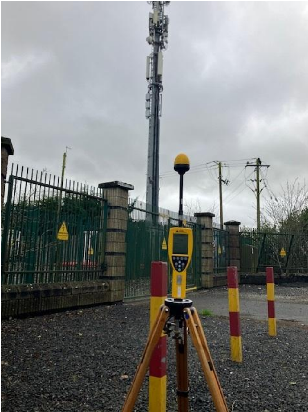
Photo 1. Broadband Measurement location looking towards antennas
