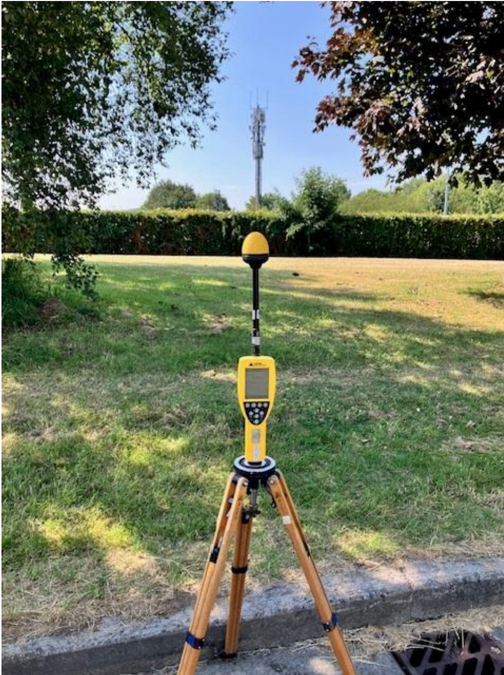
Photo 1. Broadband Measurement location looking towards antennas
