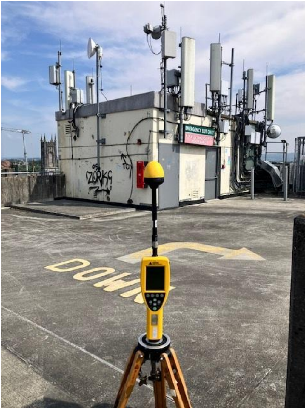
Photo 1. Broadband Measurement location looking towards antennas
