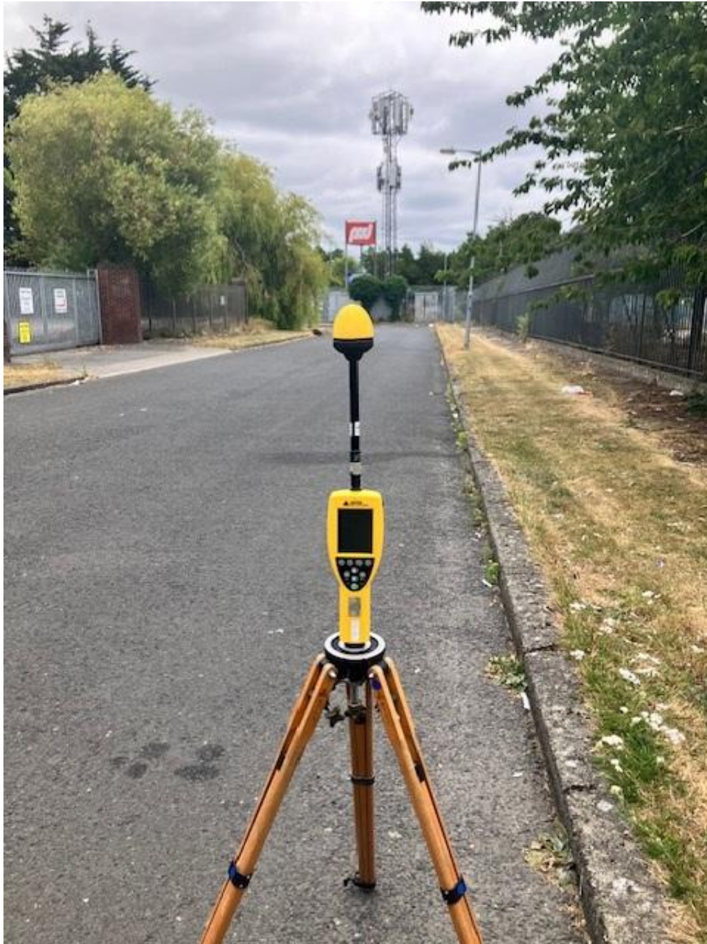
Photo 1. Broadband Measurement location looking towards antennas
